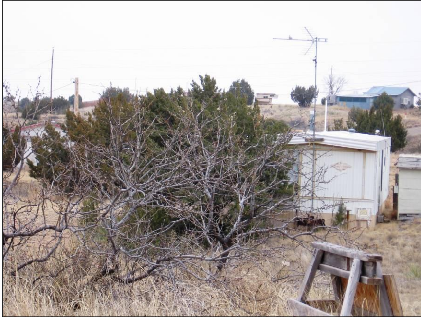
Figure 5.3. Structure requiring defensible space and fuels mitigation.
